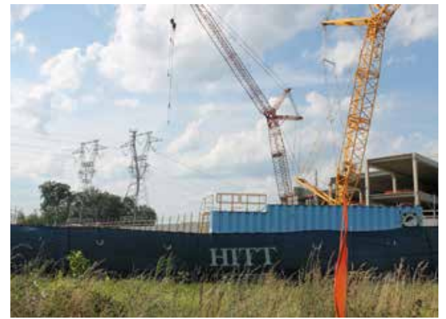
Data center construction as seen from Hiddenwood Lane.
